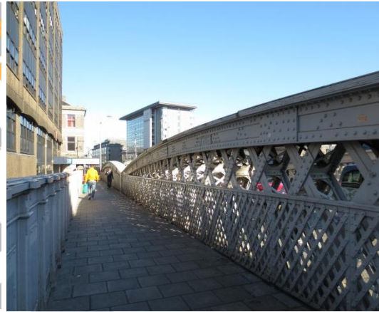
Figure 7: Guild Street Bridge
